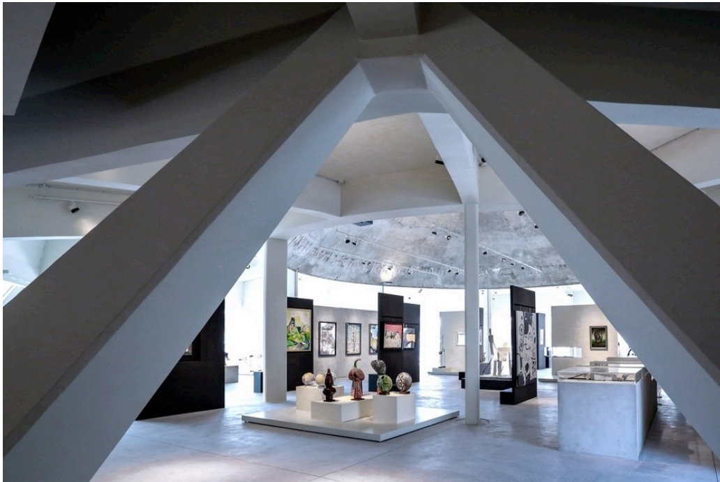
The Flying Saucer's echoing dome rests on slender columns and a series of triangulated, interconnected concrete beams. Victor Besa for The National
